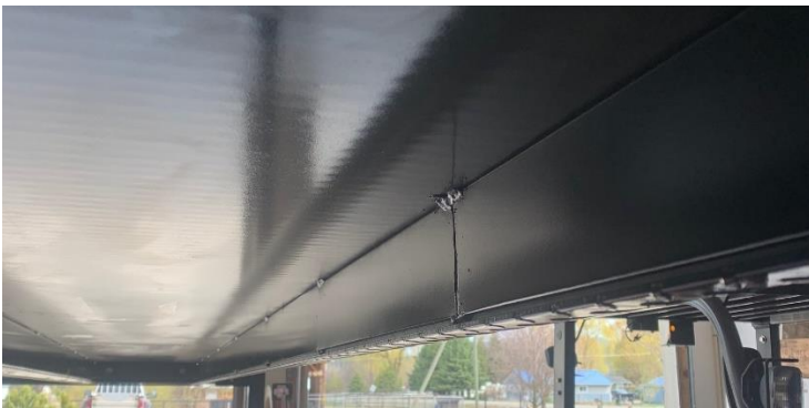
Welded on steel doubling for extra strength, ramps and Xbars
