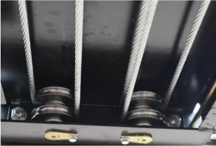
Cables and pulleys under the main runway
